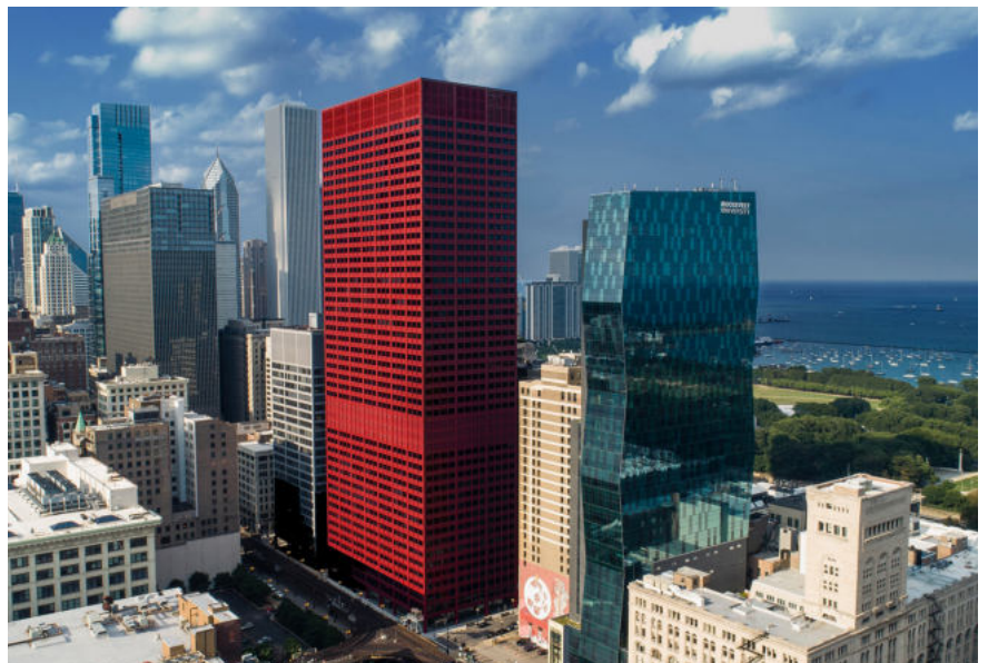
„BIG RED“ PRIME OFFICE TOWER – CHICAGO
